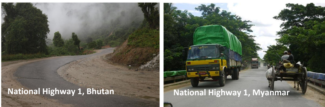
Figure 1-2: National Highway 1 in Bhutan and Myanmar
